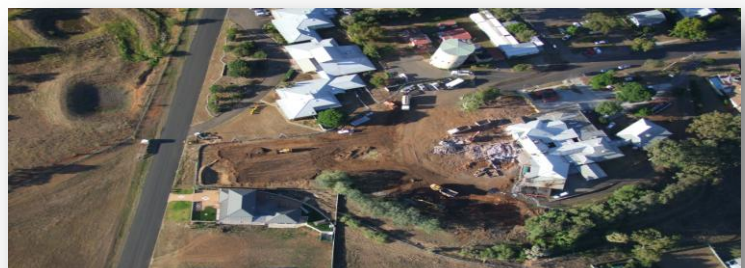
HealthOne Manilla construction site
