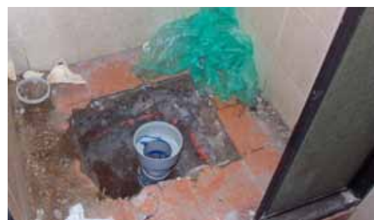
2. Leaking showers are stripped, waterproofed and rebuilt.
