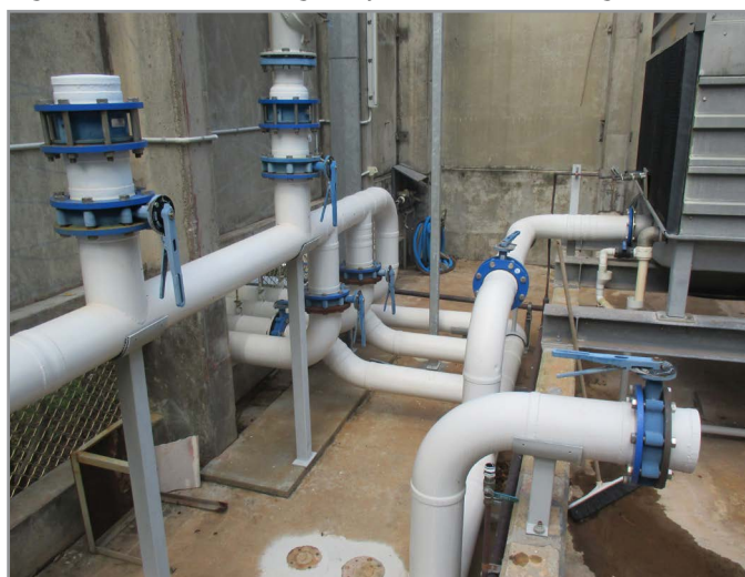
Figure 5.1-1: Two dead legs (top left and bottom right)
