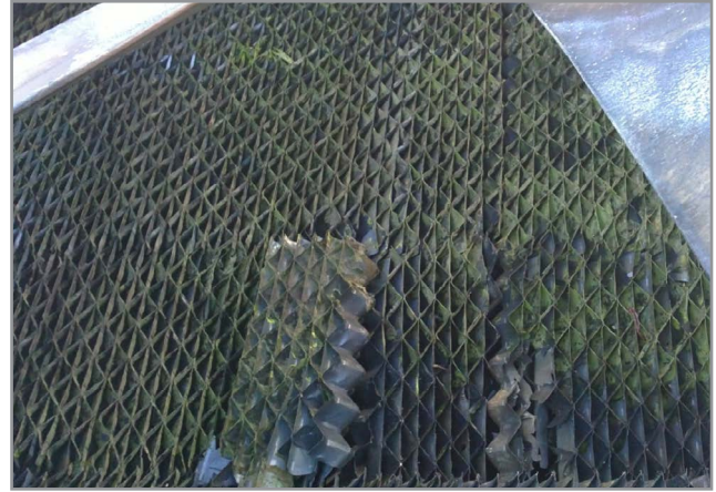
Figure 5.4-3: Damaged drift eliminator sections with algal build up
