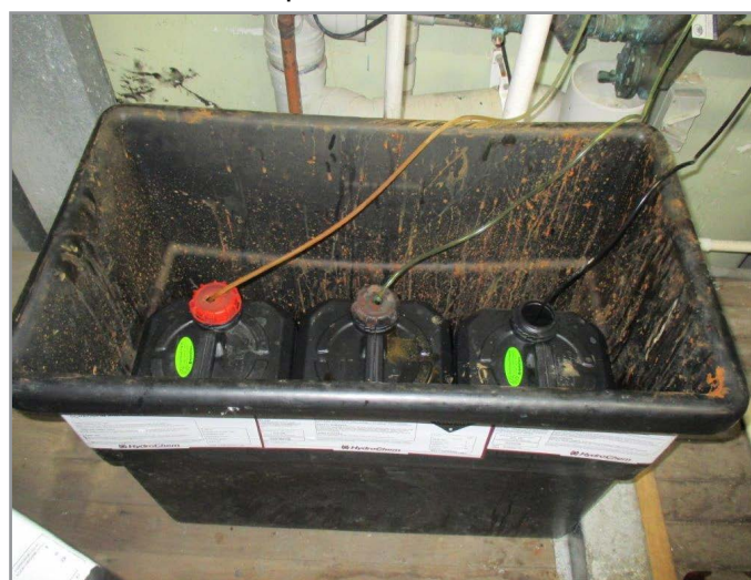
Figure 5.3-5: A bund container that may compress dosing tubes when the lid is replaced
