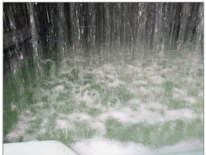
Figure 5.1-4: Even fall of water across basin area suggests fill passages are clear
