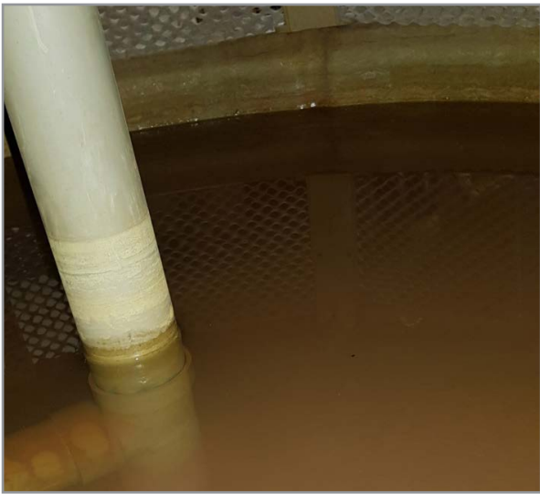
Figure 5.3-1: Cloudy or discoloured cooling water can indicate poor water cleanliness or insufficient cleaning and servicing
