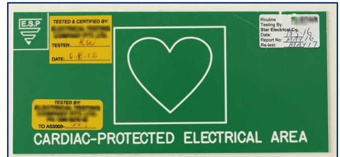
Figure 2-6. Signage denoting electrical protection
