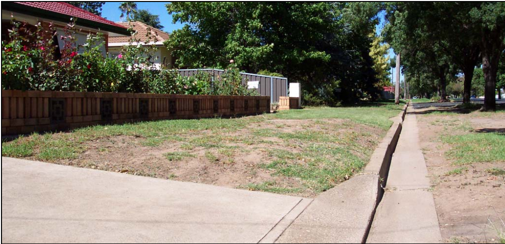
Figure 7 Uneven grass footpath in Raymond Street, Wellington, New South Wales
