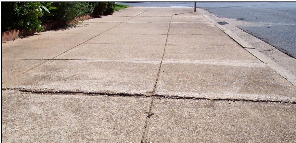
An uneven concrete footpath in Lee Street, Wellington, New South Wales
