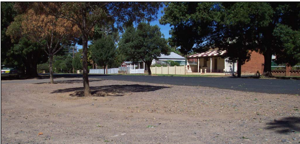
Figure 8 Unsealed road in Raymond Street, Wellington, New South Wales
