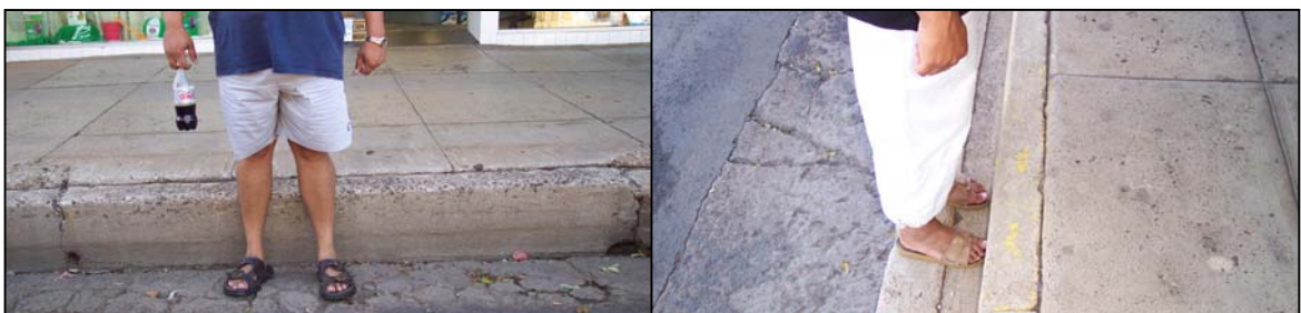
Figure 10 Kerbing on the eastern side of Nanima Crescent, Wellington, New South Wales
